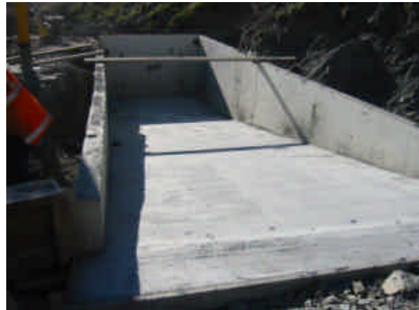
Concrete sump where the workers received their burns
